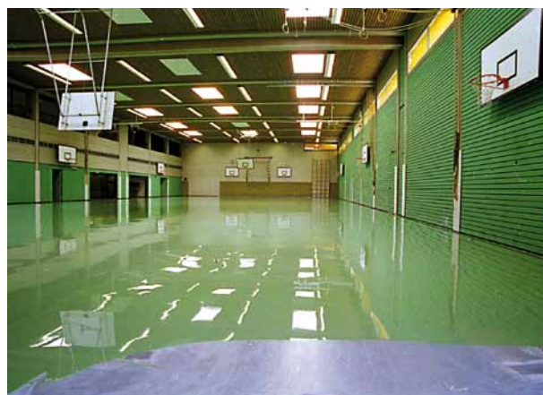
Casting and levelling the polyurethane wear layer.
